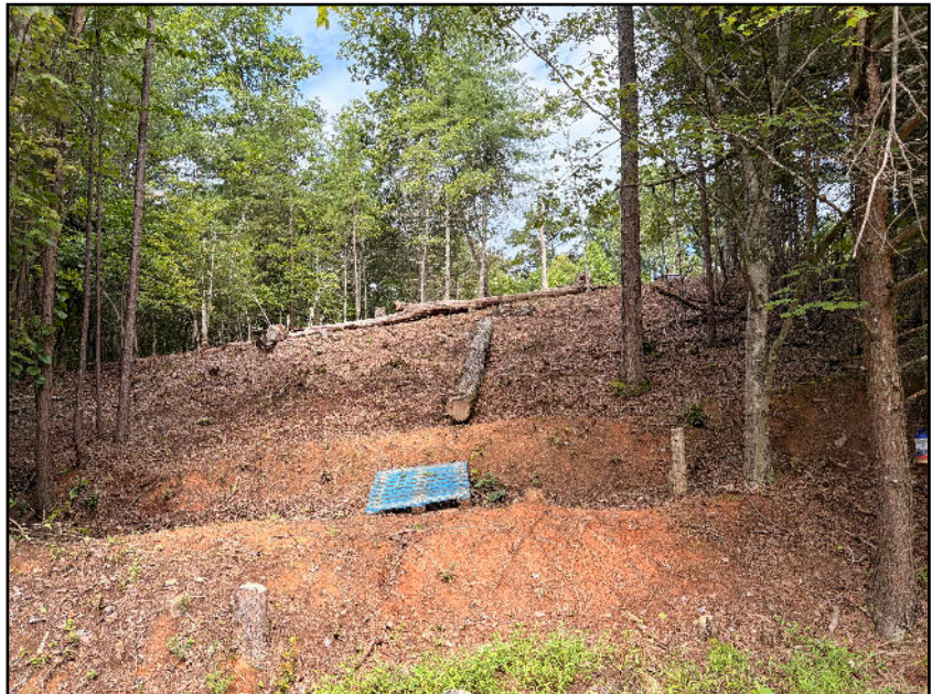
Figure 5: Land clearing for the new Terrace.
